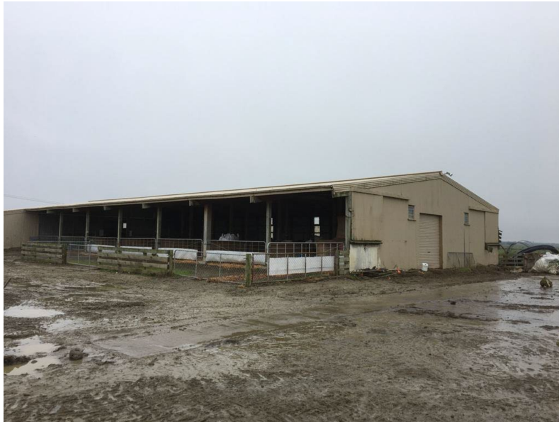
Figure 2: Calf shed with drainage installed to prevent large puddle forming
