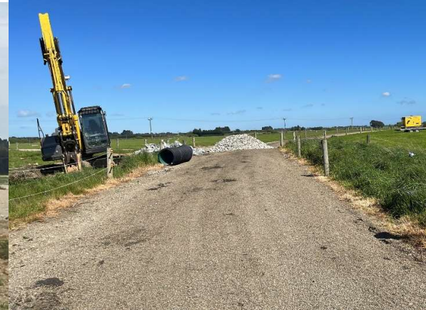
Flood repairs to the culvert
