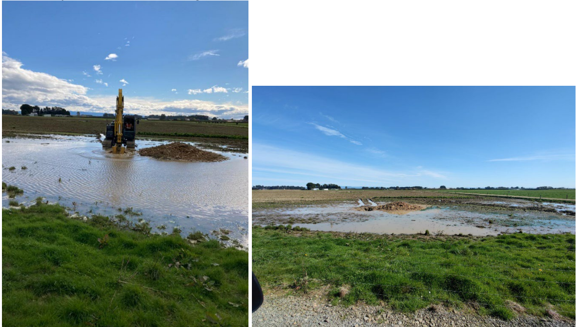
Figure 7: Remedial work out from the dairy
