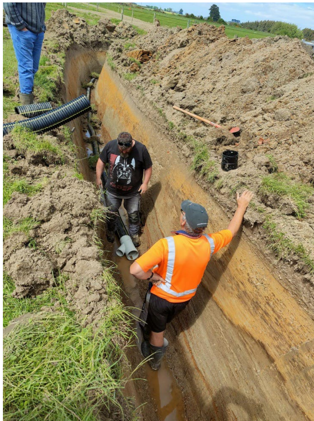
Figure 4: Contractors putting in drainage to get the drainage system operating efficiently
